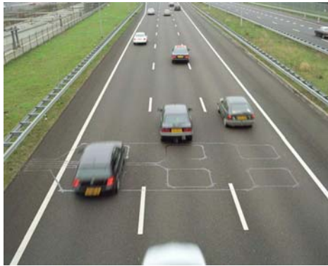
(a) Photo of a dual ILD setting for 3 lanes [36]
