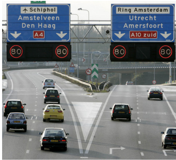
Figure 4.3: Dynamic Route Information Panel (DRIP)
